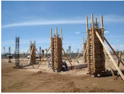
Figure 2. Falsework of concrete columns.
