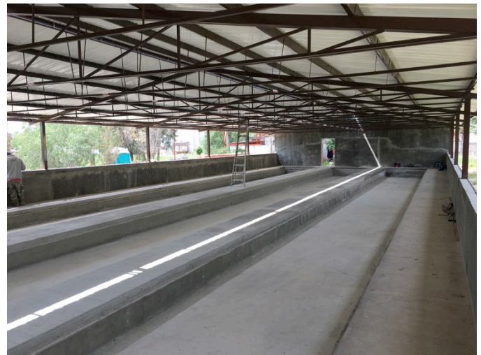
Storage pit used as drainage in a maternity shed for sows.
