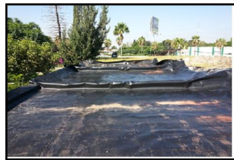
Figure 5. Picture of geomembrane colocation.
