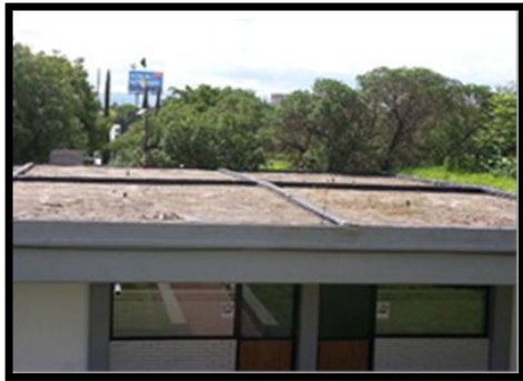
Figure 6. Colocation of the substrate.
