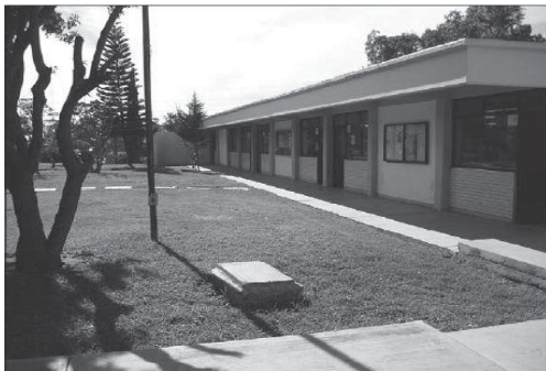
Figure 1. Classrooms of the studied building, south view.
