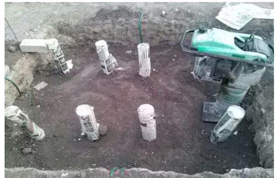
Fig. 7. Compaction of the expansive soil with the vibrator compactor.
