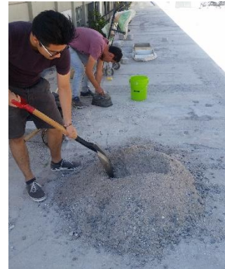
Fig. 6: Mixing sand and gravel.
