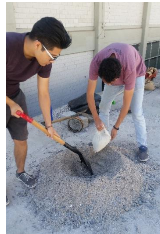
Fig. 7: Mixing concrete.
