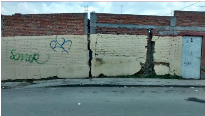
Fig 1. Subsidence, Social consequences of an induced disaster San Antonio street, Neighbourhood San Pablo [15].
