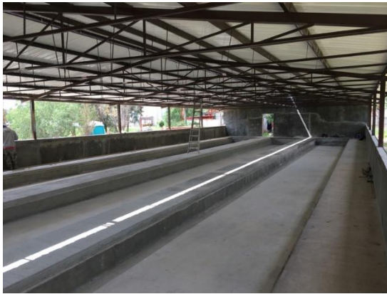
Figure 2. Storage tank drained by gravity used as drainage in a house for sows in maternity stage in the area of El Márquez, Querétaro.
