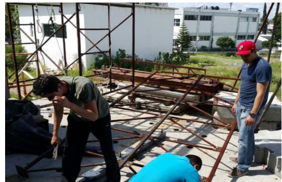
Image IV. Fixing the first lightweight panel.
