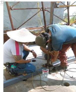
Image IX. Correction of drilling.
