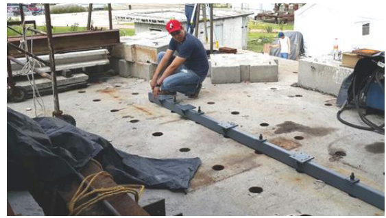
Image II. Secondary base structure for fixing the panel. (5).
