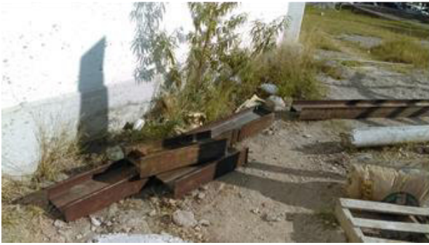
Image X. IPR profiles cut to the required measurements.
