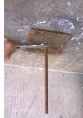
Image III. Placement of stud bolts to fix panel base.
