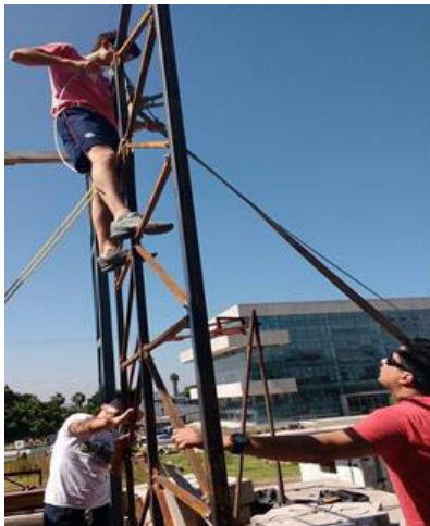
Image XII. Leveling and tensing the panel.
