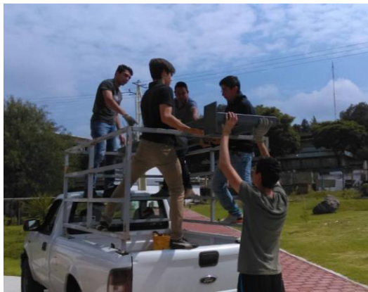
Image I. Move of auxiliary structure for lightweight panel.
